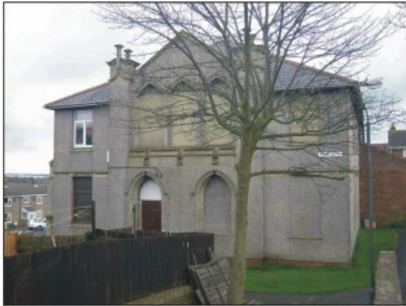
The Former Wheatley Hill (Primitive) Methodist Chapel, west frontage
