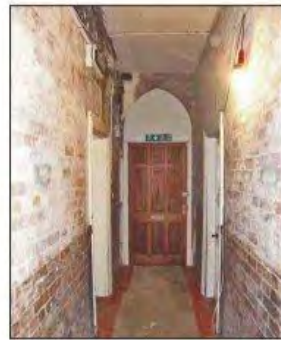
View westwards along early 20th century schoolroom passage, towards arched entrance doorway.
