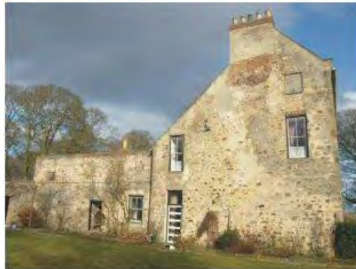
Thornley Hall, west frontage
