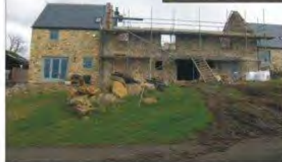
'Sutton Newbold' following removal of roof timbers
