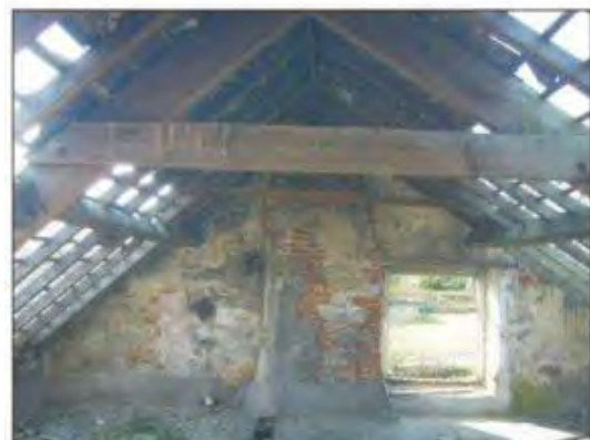
View of west gable end at roof-space level.
