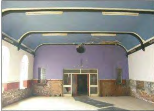
Interior original chapel hall, looking south.
