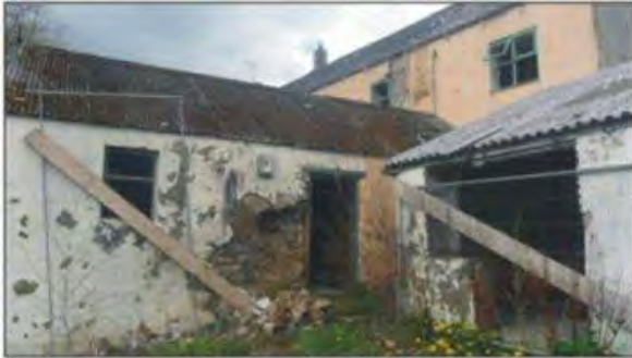
The farm-buildings, NW corner of western yard
