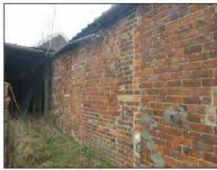
Part of the south range - note blocked arch.
