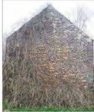
East elevation of the detached North-East (NE) range.
