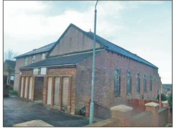
The south and east frontages viewed from SE.
