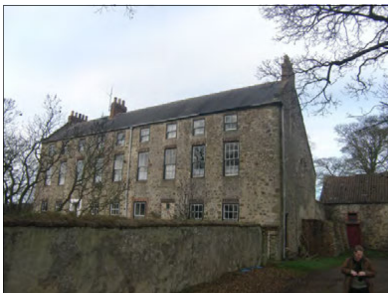
Illus. 10.19: View of Thornley Hall from the SE. The hall was probably built c.1700 but may contain earlier fabric.
