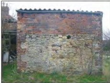
South elevation of outbuilding west of the farmhouse incorporating magnesium limestone rubble in its fabric.
