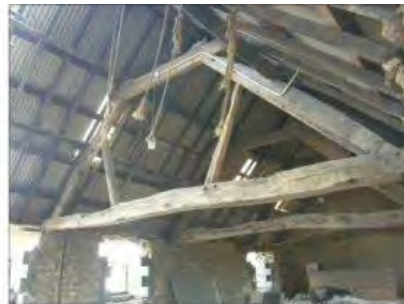
'Sutton Newbold' roof structure.
