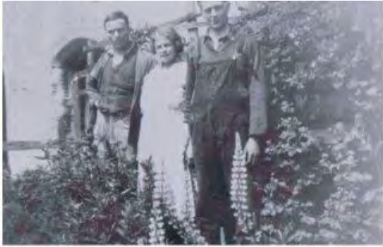
[Illus. 17] South cross-passage doorway in 1947
