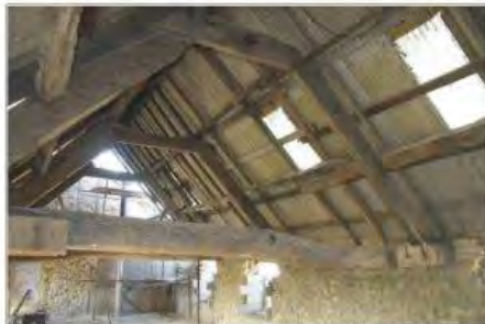
'Sutton Newbold' roof viewed from the east.
