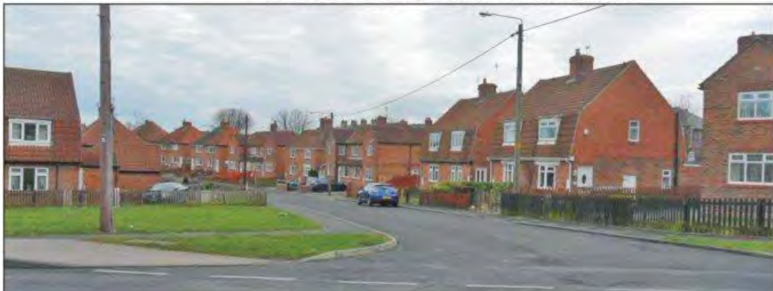
(Below) Morris Crescent, Thornley - typical mine worker's residential development of the later period.
