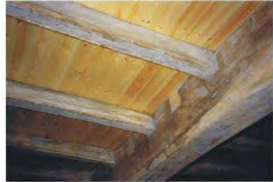
[Illus. 25] Parlour beam repaired
