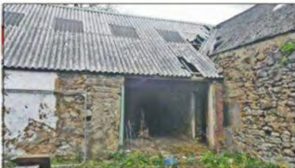
The south elevation of the Engine House.
