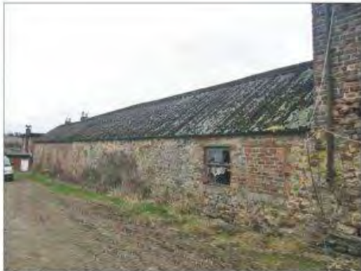
North elevation of the south range, viewed from the north-west
