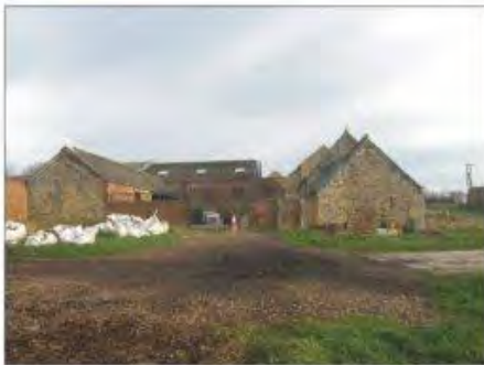
The western range of barns around yard.
