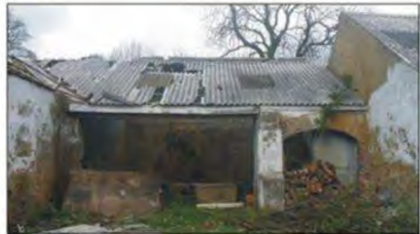
The farm-buildings, north range of eastern yard.
