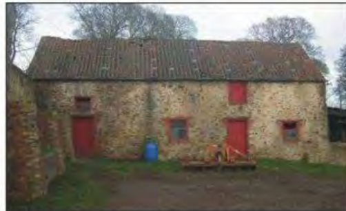
Thornley Hall, south frontage of barn.
