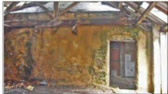
Internal east elevation of the Engine House and entrance to barn.
