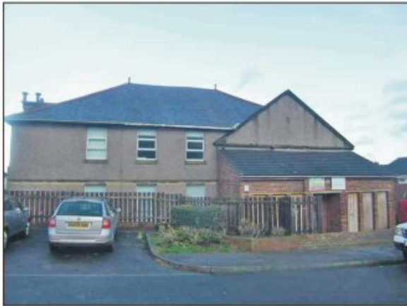
The south frontage and modern porch addition.
