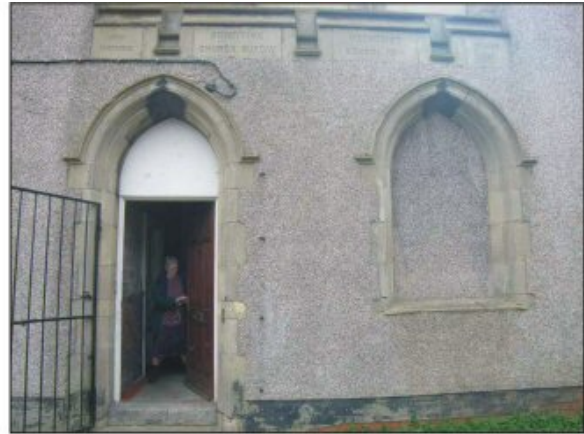
Detail of west frontage doorway and inscriptions.
