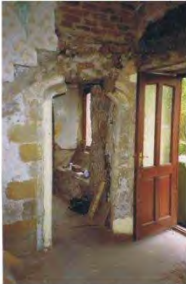
[Illus. 28] Traces of former stairs above parlour door next to present entrance
