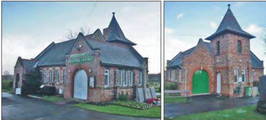
The Wheatley Hill cemetery former chapel of rest (now Heritage Centre).
