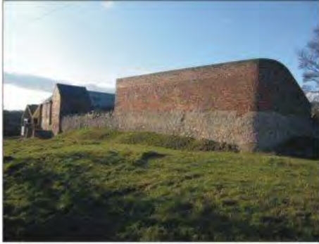
Thornley Hall farmyard wall
