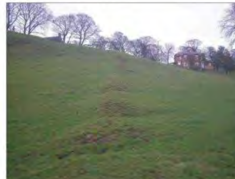
Earthwork on meltwater channel valley side south of Thornley Hall farm cottages
