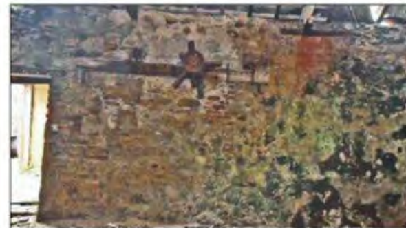
Remains of machinery on internal west wall of the long barn.
