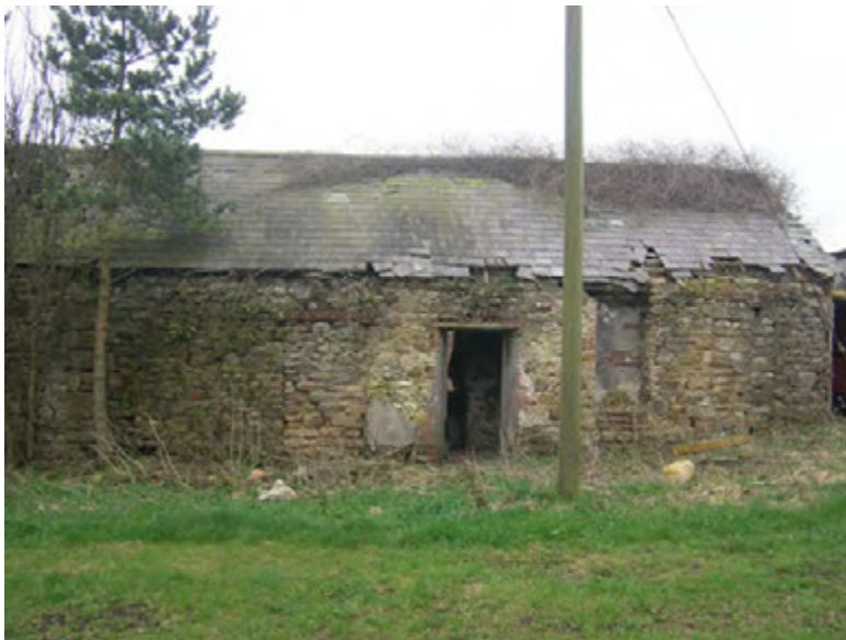
The west end of the north range of Wingate Grange Farm, showing the earliest fabric associated with the large quoins in the north wall.
