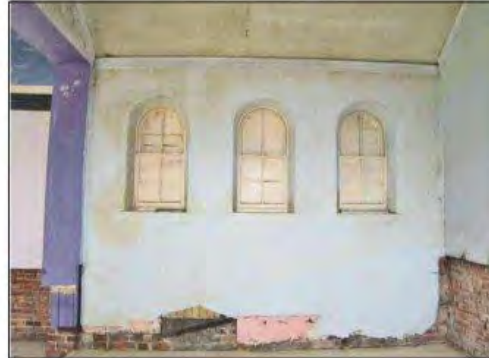
Interior west chancel wall.
