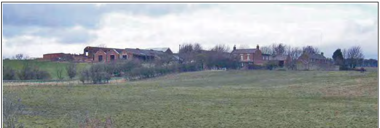
Wingate Grange Farm viewed from the south-east.
