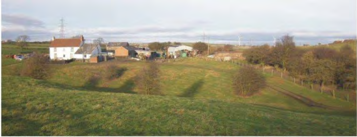
White House Farm viewed from the south.
