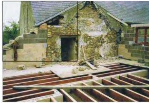
[Illus. 8] Rear Wing first floor and roof-space levels
