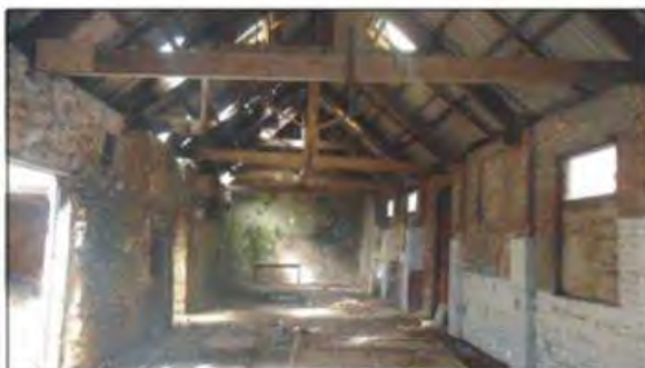
Long eastern barn interior viewed looking north.
